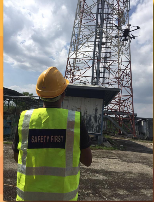
Drone Inspection Operation + Overall Tower Profiling 20 minute flight per inspection work
